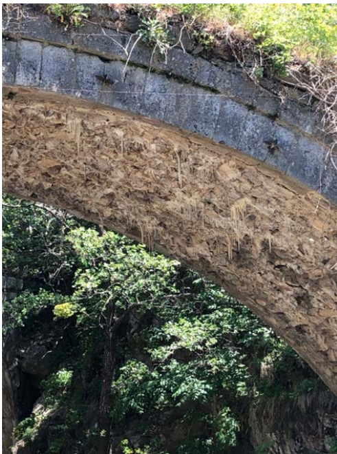
Fig. 8a, 8b: Views of Dušan's stone bridge
