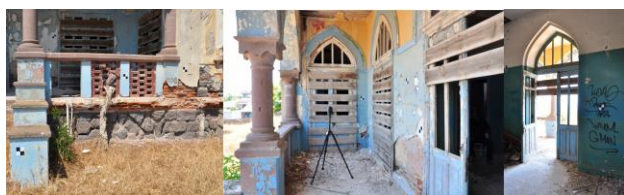
Figure 3: Views from parts of the building that were scanned and the use of targets for the data capture.
