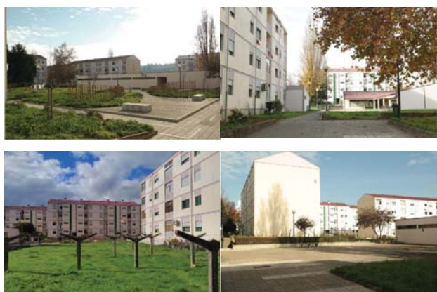
Fig. 3 – Existing situation: (top-left) north entrance; (top-right) view to the commercial 1 floor building; (bottom-left) clotheslines; (bottom-right) southwest entrance.
