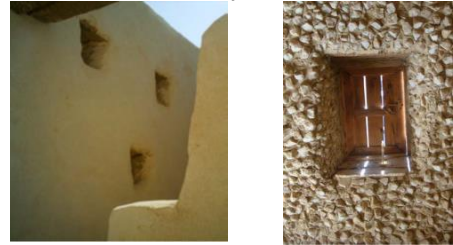
Fig. (28) Small windows imbedded in the thick walls.
