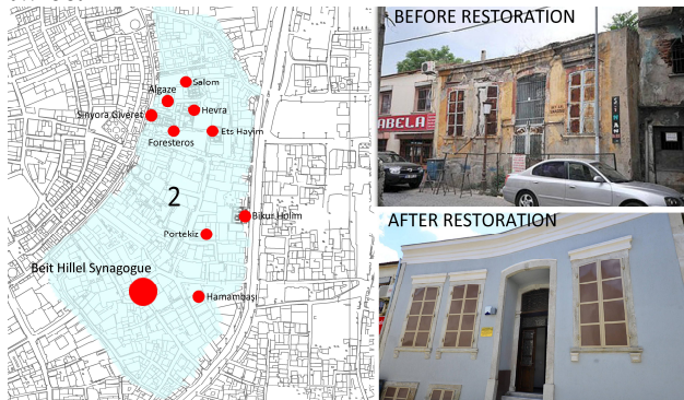
Fig. 11 Location of 2. Sub-region and Beit Hillel Synagogue before and after restoration [9]
