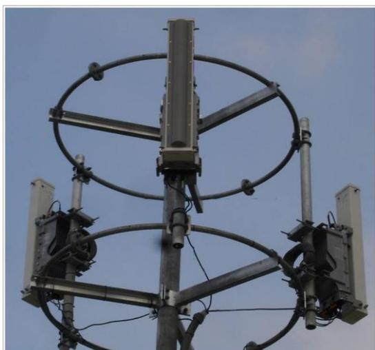
Figure 18. The 3-sectors BTS antenna installation.
