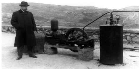
Fig. 2 Lardarello 1904: Principe Piero Ginori-Conti is shown here with his device that produced the first-ever electrical energy from geothermal energy.
