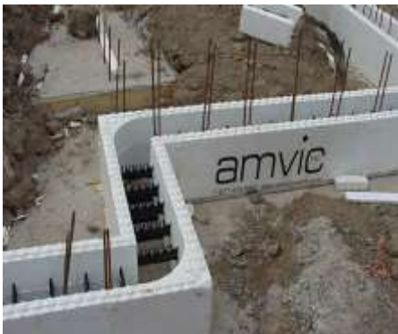
Fig.40: Short corner made of 90° forms with a running bond
