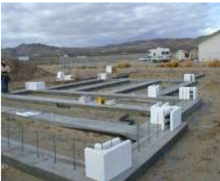
Fig. 29: Placing corner block first
