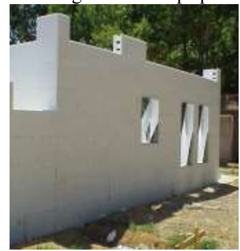
Fig. 21: Continue installing block courses.
