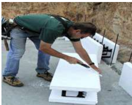
Fig. 31: Cutting the final block for a wall section.
