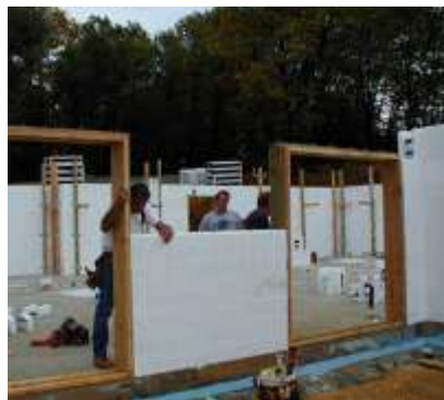
Fig. 20: Install window and door bucks.
