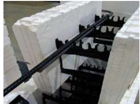
Fig. 18: Install horizontal reinforcing steel and lap splicing
