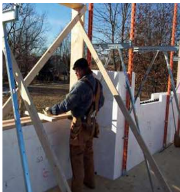
Fig. 22: Install alignment and bracing around the interior of the perimeter wall.
