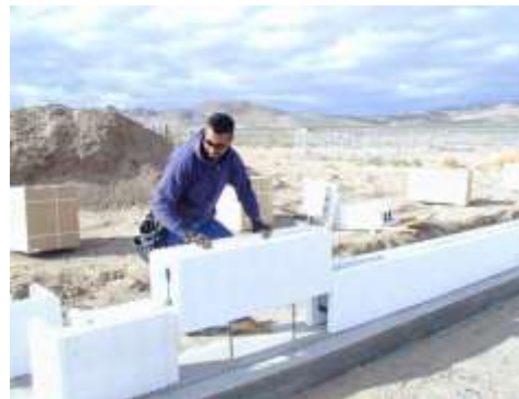
Fig. 30: Placing straight blocks
