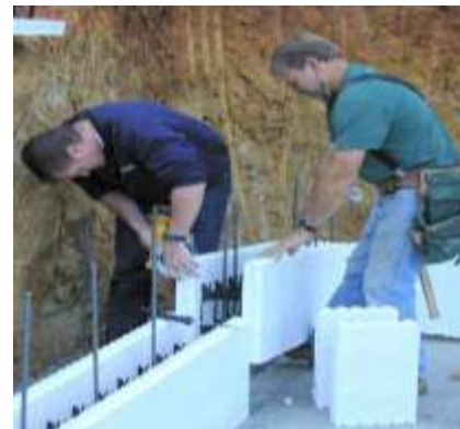
Fig. 32: Fitting the cut block in place.
