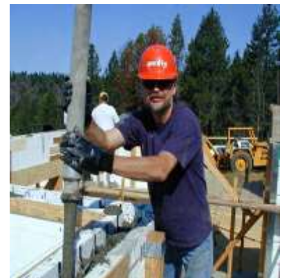
Fig. 24: Install vertical reinforcing bars after top course of blocks.
