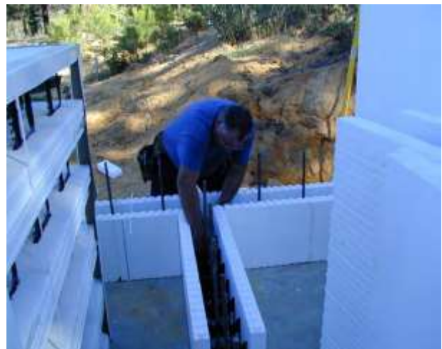
Fig. 47: Install horizontal reinforcing steel bars as each course is laid
