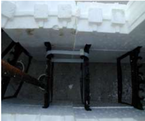
Fig. 33: Using zip ties to tie the first course of blocks together.
