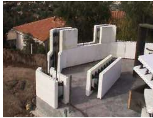
Fig. 35: Reversing 45° corner blocks for bay window
