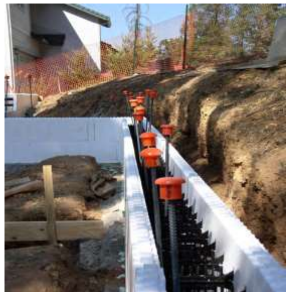
Fig. 27: Plastic mushroom caps on protruding steel bars
