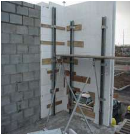
Fig. 38: Bracing corners
