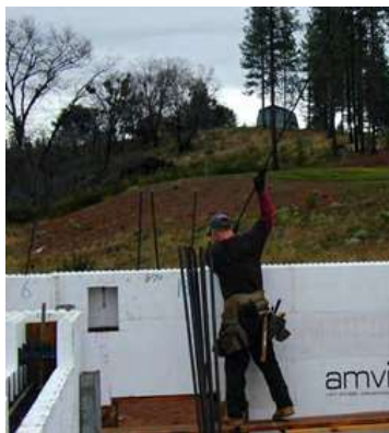
Fig. 23: Install vertical reinforcing bars after top course of blocks.
