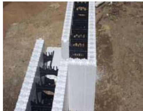
Fig.41: Using cut-off pieces to close the open ends and create a corner
