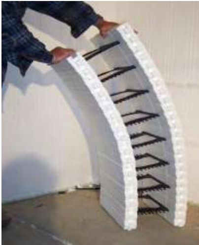
Fig. 44: Bending and securing the radius form into place
