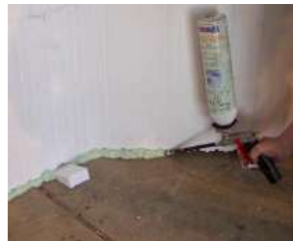
Fig. 37: Gluing an unshaven course to the footing/slab
