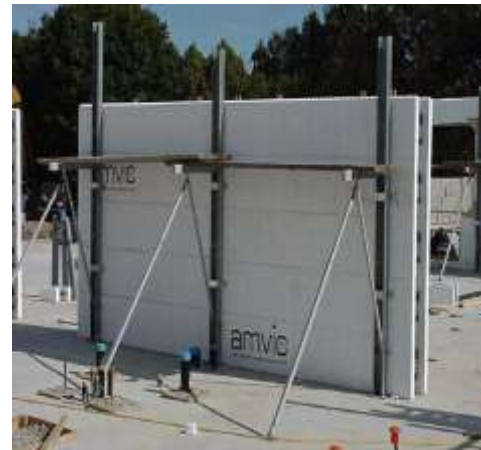
Fig. 39: Platform and scaffold planks.
