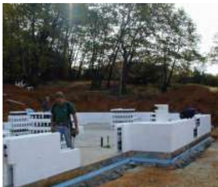
Fig.19: Install second course of blocks.
