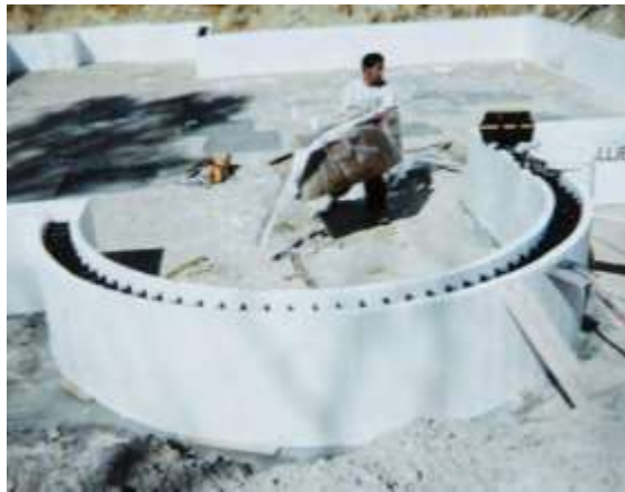
Fig. 45: Several courses of radius blocks installed
