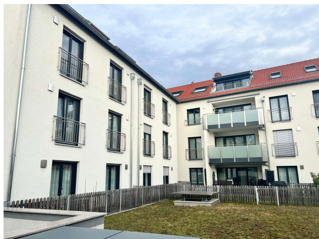
Figure 2 Multifamily House in an Urban Area (house 1,2)
