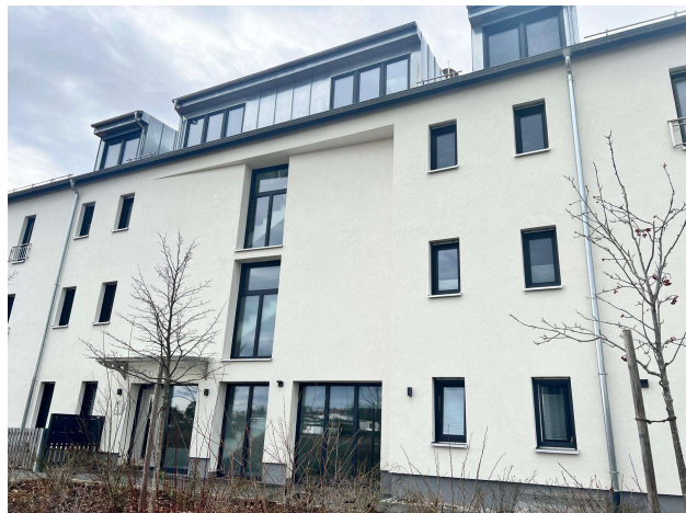
Figure 1 Multifamily House in an Urban Area (house 1)
