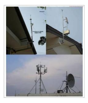
Figure 17. The 3-sectors WBBN's antenna at Health center and MSMC building.
