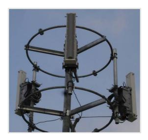
Figure 18. The 3-sectors Wi-MAX BTS antenna installation.
