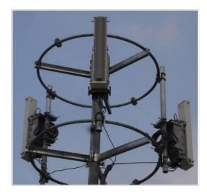
Figure 18. The 3-sectors BTS antenna installation.
