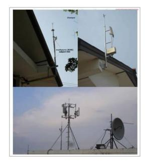
Figure 17. The 3-sectors Wi-MAX's antenna at Health center and MSMC building.
